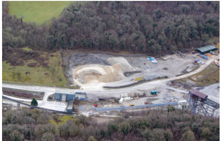
Existing site, looking South
