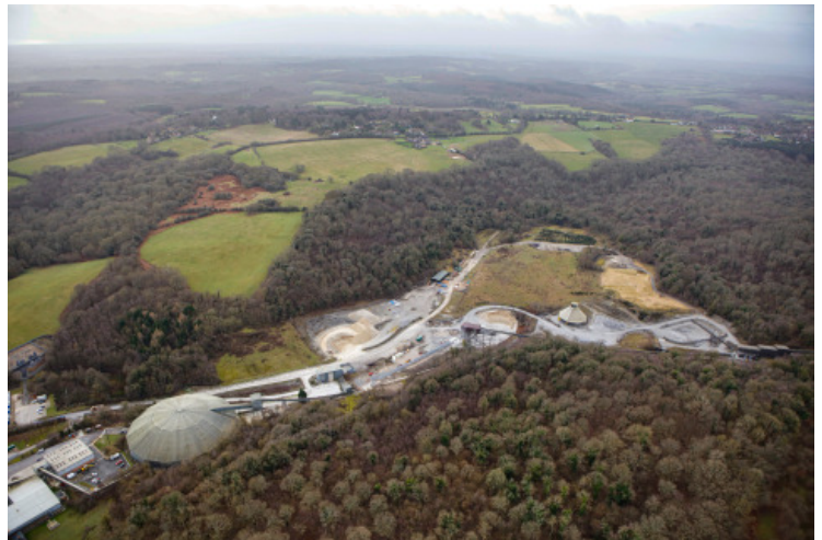
Existing site, looking South
